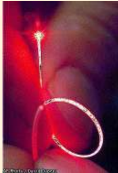
A single strand of optical fiber can handle 5 million telephone Photo by David Duprey
